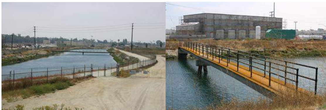
Figure 7-4. Existing Footbridge over Haynes Channel
