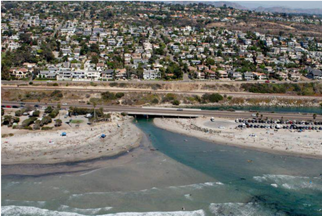
Figure 7-142. Example Low and Short Bridge Over Soft-Bottomed Wetland Area Highway 101 Over San Elijo Lagoon in Encinitas, CA
